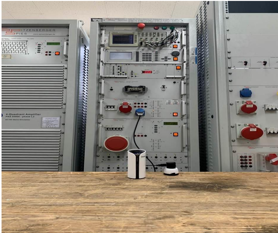
Photo of test setup for Harmonic Current Emissions
